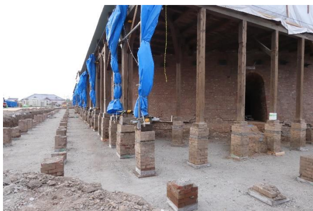
輪窯外周の掘削
